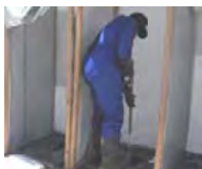
Figure 40. Water jetting to liquefy trench latrine wastes
