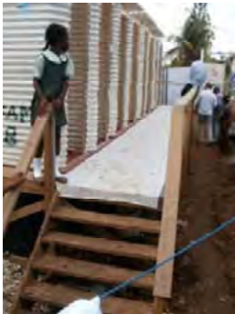
Figure 4. Entrance platform for a raised latrines in ?? camp
