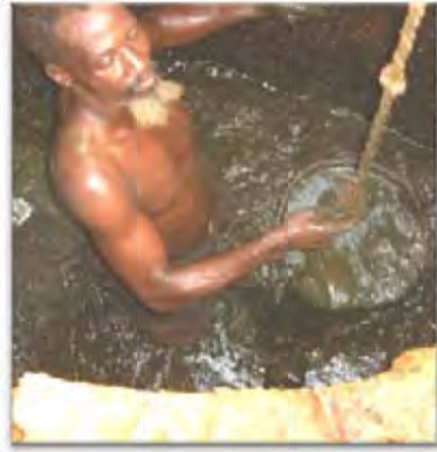
Figure 47. Manually emptying a pit latrine
