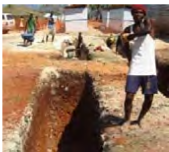
Figure 19. Digging trenches for toilets
