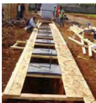
Figure 20. Installing squatting pans over a trench
