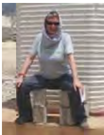
Figure 17. Block pedestal for disabled users
