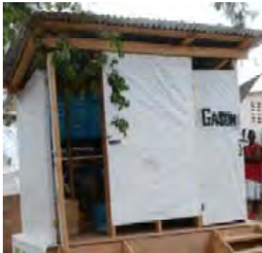
Figure 6. Timber framed door with simple internal lock on a urine diversion toilet in ?? camp
