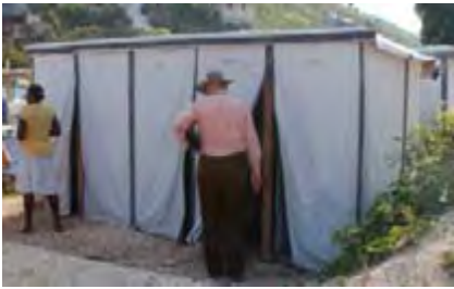
Figure 5. Sheeting doors on a trench latrine in ?? camp
