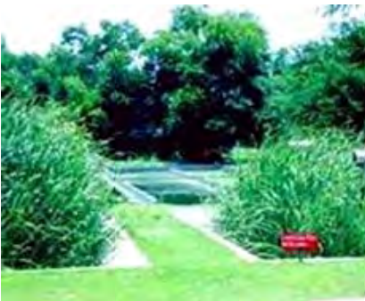
Figure 63. Established constructed wetlands
