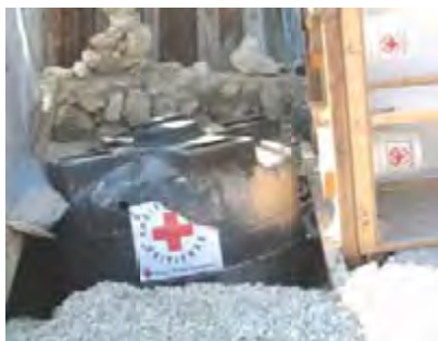
This tank was buried but floated after rain. Note 4 holes in top
