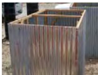
Figure 22. Prefabricated trench lining in ?? camp to support weak soils
