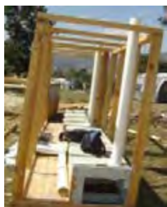
Figure 21. Pedestal toilets for trench latrine under construction
