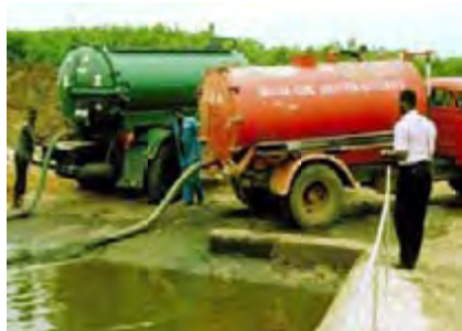
Figure 59. Discharging faecal sludge into WSPs
