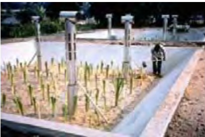
Figure 61. Wetland under construction
