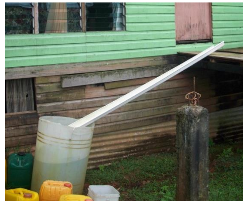
Image 5.2: Crudely built DRWH system
