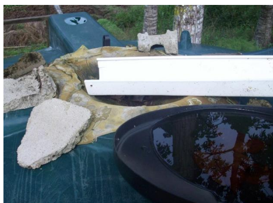
Image 4.1: Cloth screen on plastic tank
