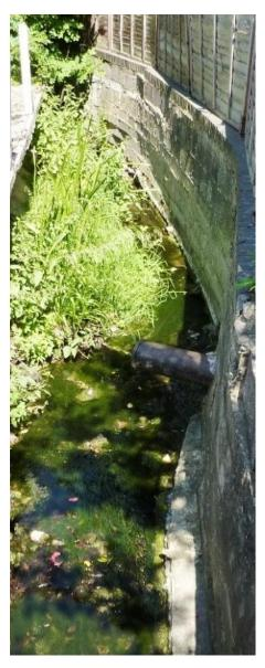
Figure 5.21 Outfall to Pontesbury Brook, presumed from highway drainage. Photograph taken by author, July 2013
