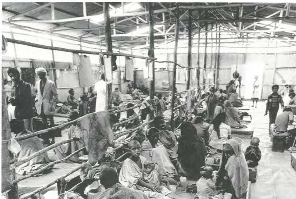
6.1.1B Korem 1985 Camp hospital. This in-patient area in a child feeding programme is housed in an RRC standard structure (4.15.3). Skylights, beds made of planks with earth infill, and plastic flooring are added improvements. (Photo: Mike Wells)
