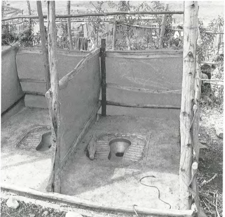
4.13.2 Bulbulo 1985 Trench latrine super-structure. The local building materials normally used are eucalyptus poles and corrugated iron sheeting. (Photo: Mike Wells)
