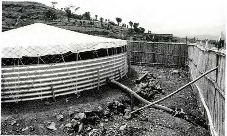
4.6.2 Bulbulo 1985 48,000 litre water tank imported as an OXFAM kit. (Photo: Mike Wells)
