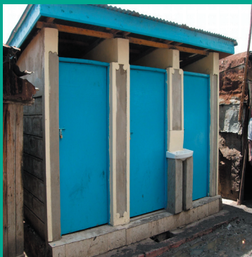
Photograph 6. Mamwika Stand-alone Toilet
