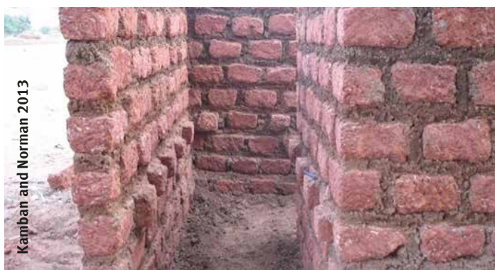
Figure 19: Latrine design with protruding bricks for support, and string for blind user to locate drop-hole.
