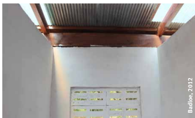
Figure 33: Transparent roof sheets to increase natural lighting
