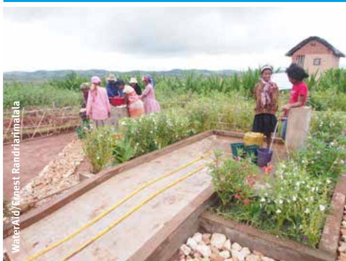
Figure 10: Example of accessible waterpoint showing wide circulation area.
