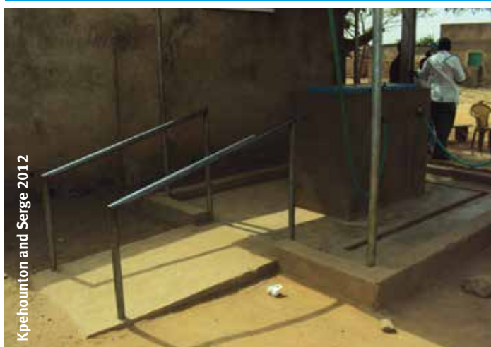
Figure 12: Waterpoint with ramp access and handrails, Burkina Faso.
