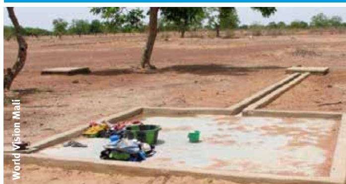
Figure 17: Design of improved laundry area, with raised sitting blocks.
