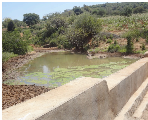
Photograph 6. Water trapped behind masonry check dam allowing slow seepage
