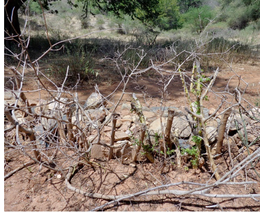
Photograph 2. Check dam: note sprouting vegetative buttresses
