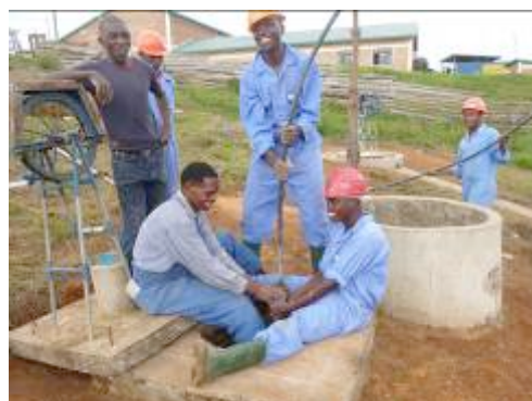
Figure 2. Making a hand dug well deeper with a tube bailer
