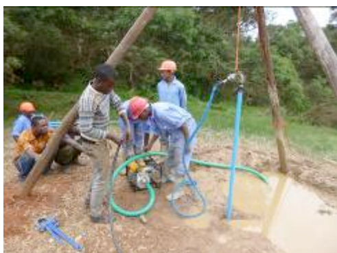
Figure 1. Manual drilling of a well of 35 m deep
