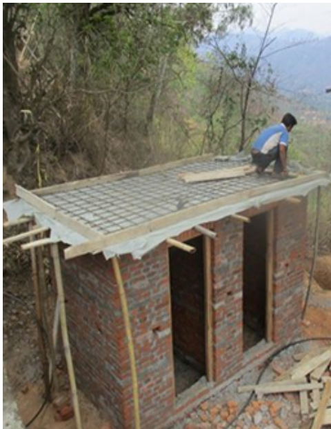
Photograph 1. WASH facilities in Hoske Health Post in Kavre district (under construction)
