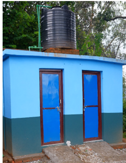
Photograph 2. WASH facilities in Hoske Health Post in Kavre district (after completion)
