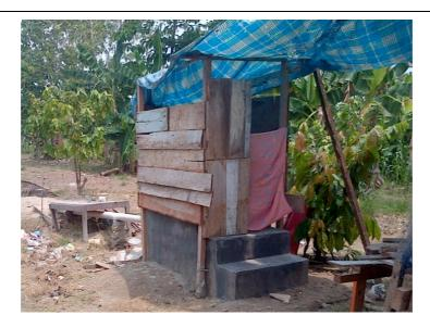
Figure 2. Example of an elevated latrine built in flood prone areas in Luwu Utara
