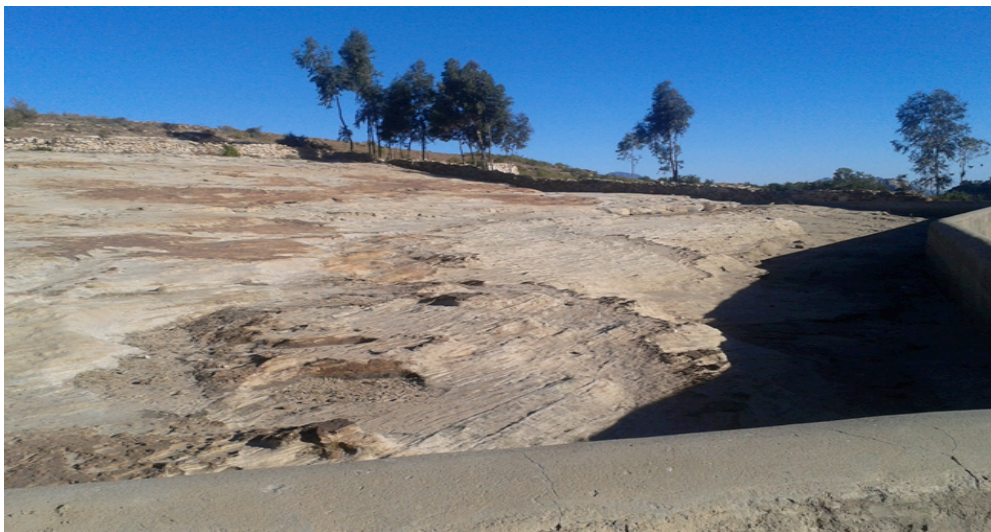
Photograph 2. Constructed structure for catchment area
