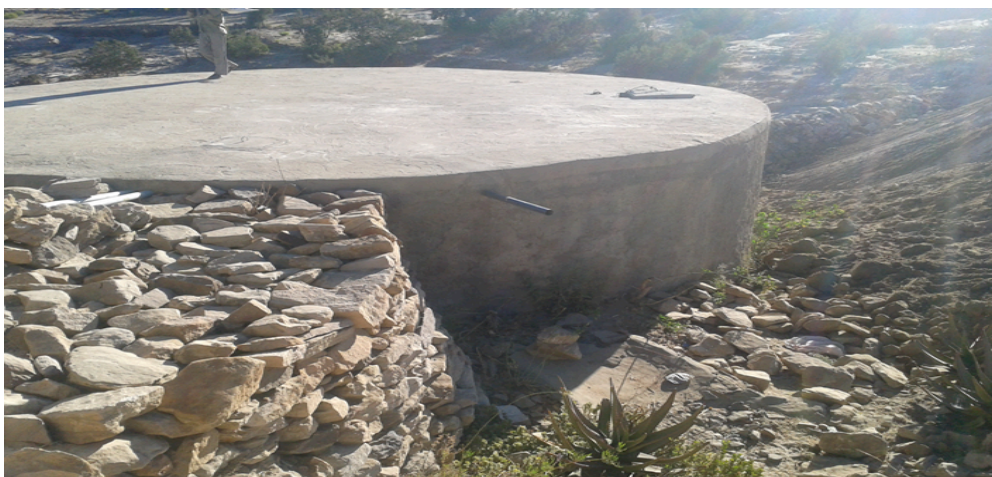
Photograph 1. Cistern for the collected water, also serves as water treatment location (if necessary)
