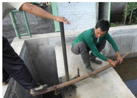
Photograph 2. Operators struggling to move SSC outlet penstock
