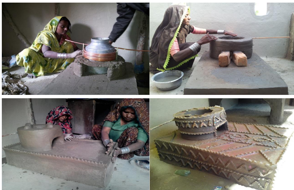
Photograph 2. Steps of the construction of the Chulli by local families
