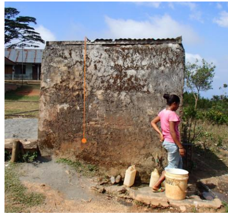
Photograph 2. Water tank showing a water level indicator
