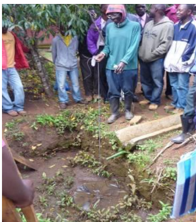
Photograph 5. Tube recharge near a family well in Njombe that had previously dried up in the dry season
