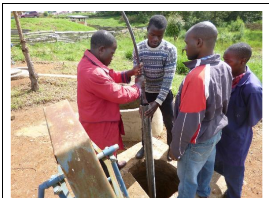
Photograph 3. Making a well deeper with the well pipe technology
