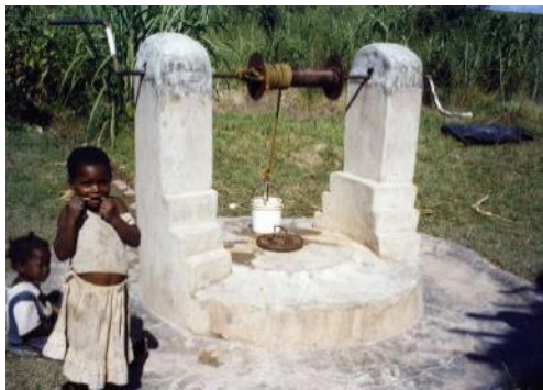
Photograph 5. Upgrading a well with a windlass like in Zimbabwe
