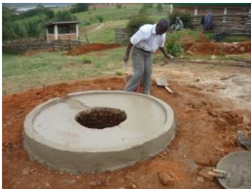
Photograph 1. Improving an open hand dug well with a well slab
