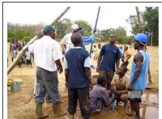
Photograph 4. Manual drilling with the so called SHIPO method
