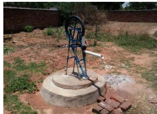
Photograph 2. An improved well with a well slab and a low cost hand pump
