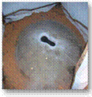
Photograph 5: Locally made dome slab, South Sudan
