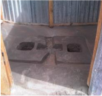
Photograph 4: Double vault urine diversion latrines, Dolo Ado, Ethiopia
