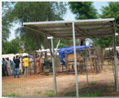
Photograph 1. Solar panels powering a submersible, Gendrassa Camp, Maban South Sudan
