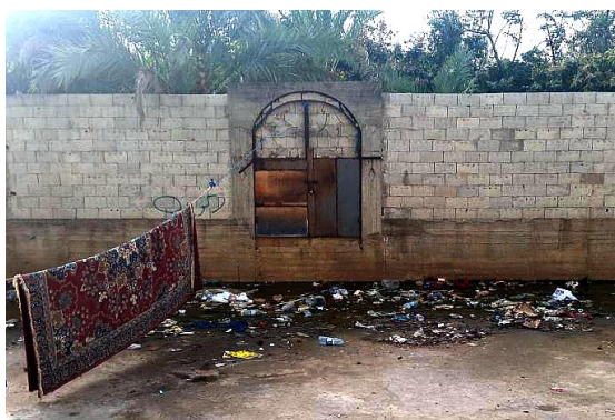
Photograph 1. Site before CWC
