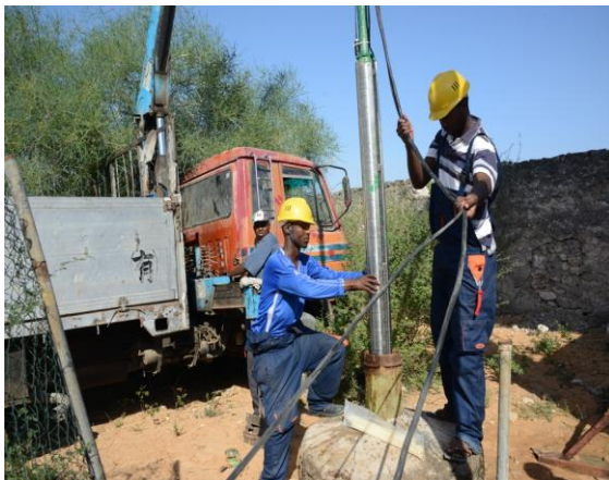
Photograph 3. Installation of the solar submersible pump in Mogadishu, Somalia
