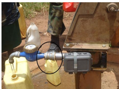
Photograph 2. Metered hand pump; Circled area shows the modification to the spout, the original spout is cut and a reducing socket is used to connect the 3/4" multi jet water meter to the spigot
