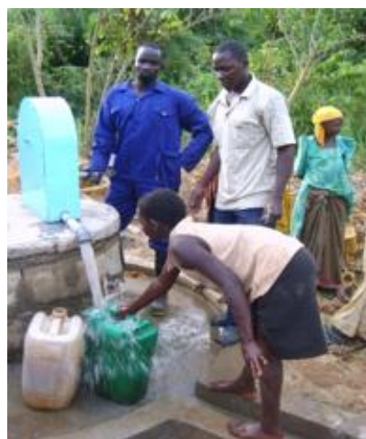
Photograph 2. The fully covered rope pump model used in Uganda until 2011.
