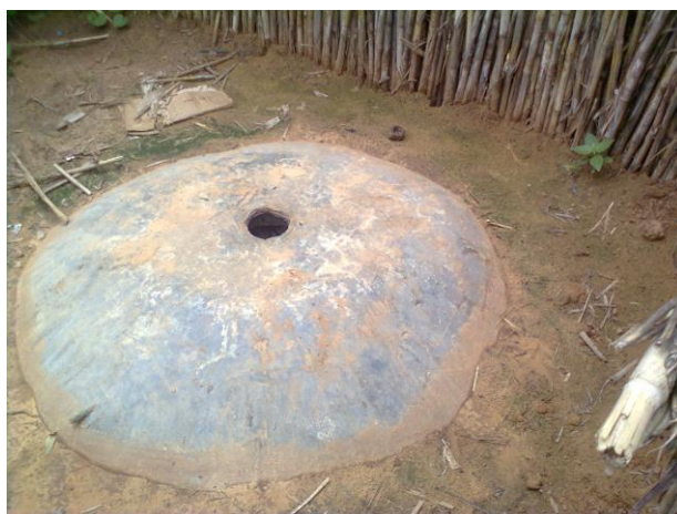
Photograph 3. The finished product of the tire type of latrine
