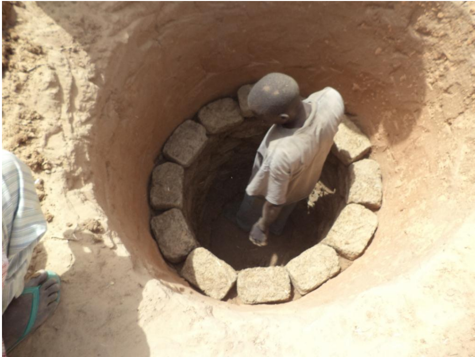
Photograph 6. The mud block type
