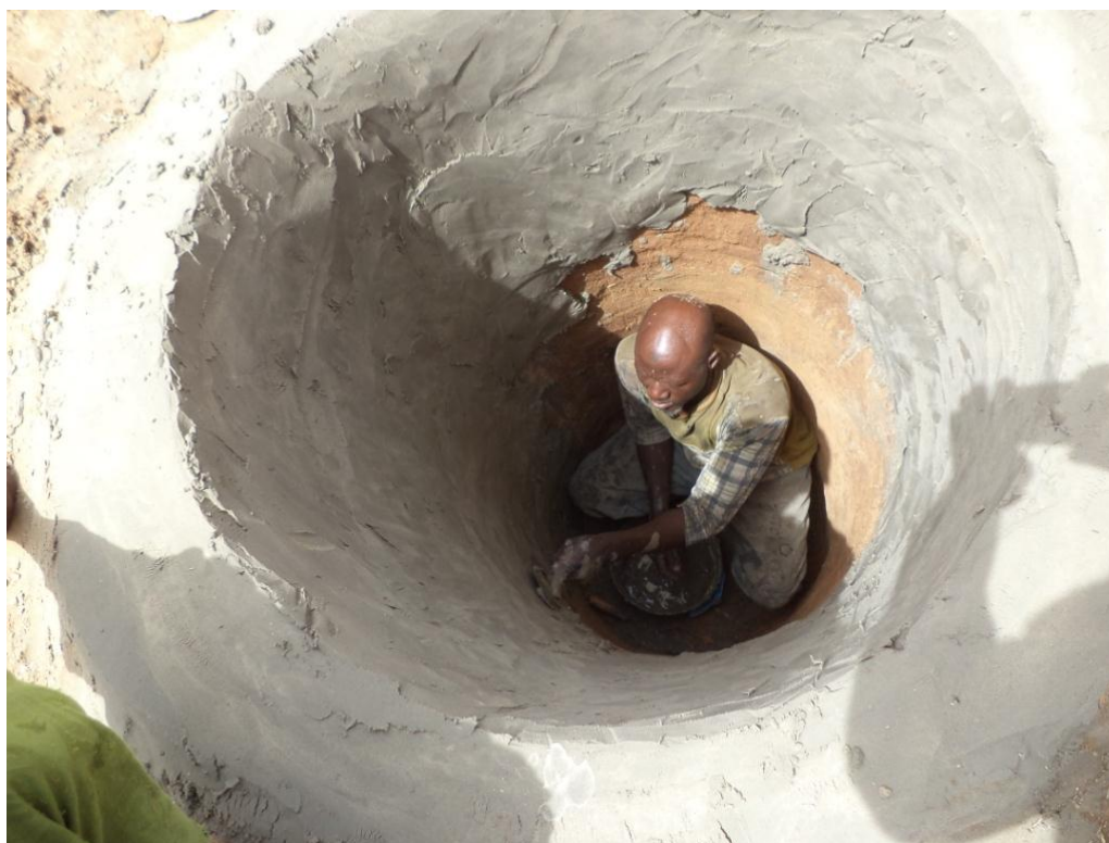
Photograph 8. Latrine walls rendered with cement to stabilise walls
