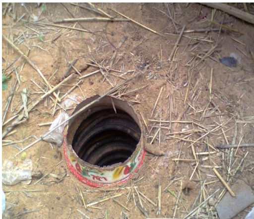
Photograph 1 and 2. The tire type of latrine under construction
