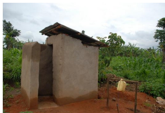
Photograph 2. One of the improved latrines constructed by a CHCs, in Gatsibo District
