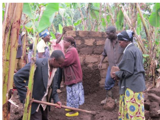
Photograph 1. Members of CHC Umucyo, Gicumbi District, constructing an improved latrine for the poorest of the community
