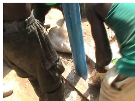
Figure 9. Installation of the gravel pack
