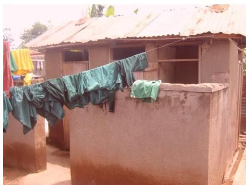
Photograph 2. Old facility where pupils had to queue (2009)
