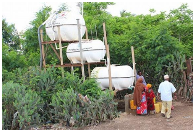
Picture 1. Three tank water treatment system in Afgoye, Somalia
