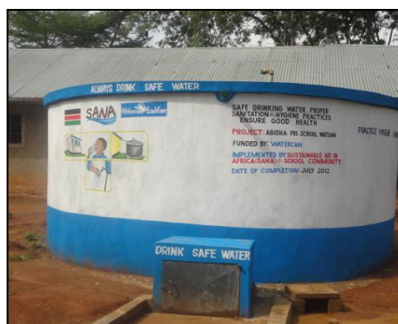
Photograph 3. Rain Water Harvesting System at Abidha PS
