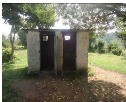
Photograph 1. Girls latrine block pre intervention at Abihda PS
