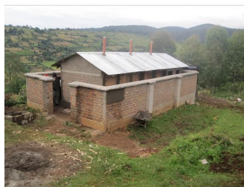
Latrines and washrooms completed
