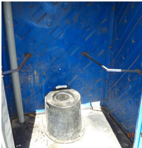
Photo 3. Cubicle with raised seat, support rails on both sides. No room to enter cubicle with a wheelchair. (Kasumba 2012)
