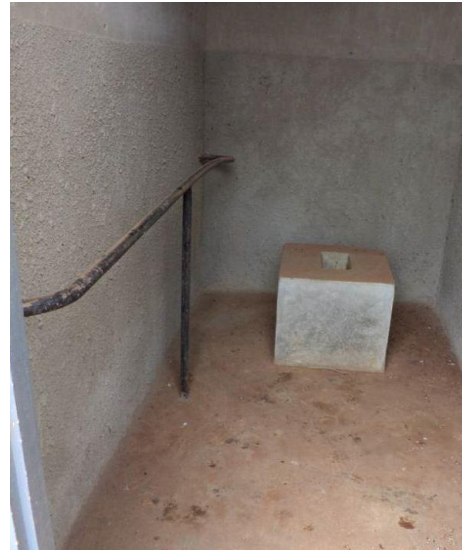
Photo 2. Cubicle with raised toilet seat and support rail. The space inside looks adequate, but the inward opening door (see photo 1) reduces the usable space. (Kasumba 2012)
