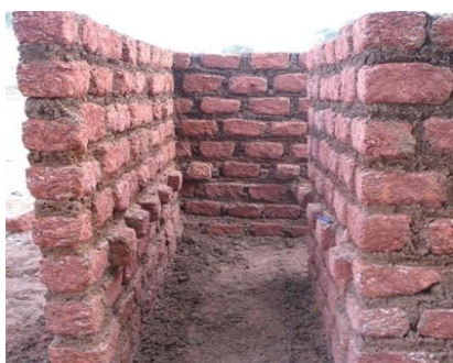
Photograph 1. Latrine handhold supports
