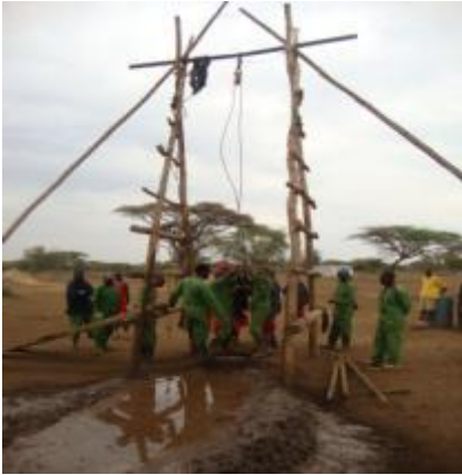
Photograph 1. Manual drilling in Kenya (IWP)
