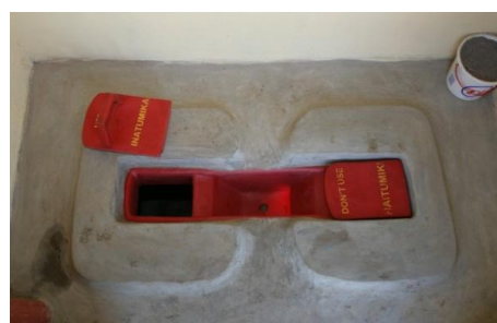
Photograph 2. Inside of household double vault UDDT with urine diversion squatting pan (with two faeces outlets) and ash bucket.
