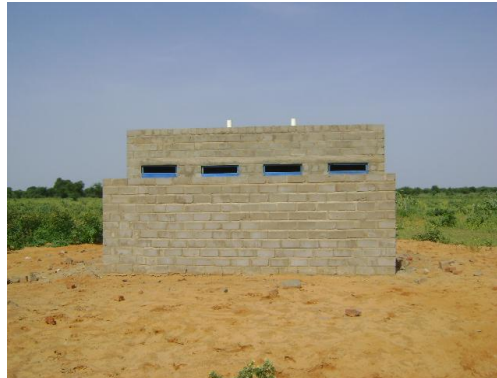
Figure 1. Latrine constructed with SSBs
