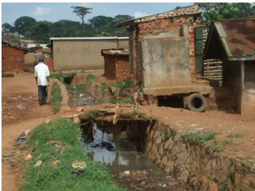
Photograph 3. Stream through area with latrine discharging into it
