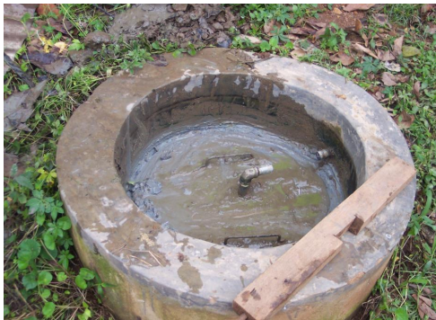
Photograph 4. Manhole cover with gas outlet
