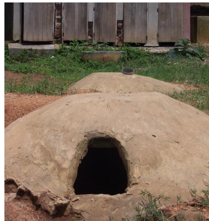
Photograph 2. Expansion chamber opening
