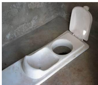
Photograph 2. Squatting toilet (glass-fibre)
