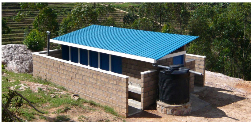
Photograph 1. UNICEF CFS toilet block
