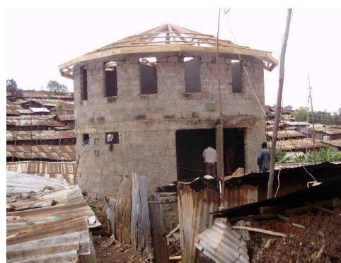
BioCentre under construction (source Umande Trust)
