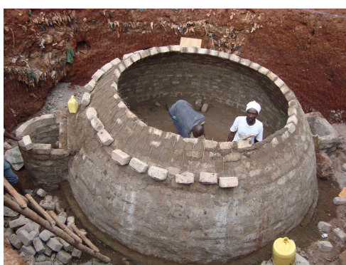
Digester under construction (source Umande Trust)
