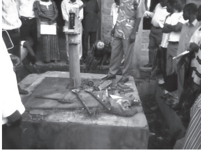
Photograph 1. Dismantling an India Mark III hand pump
