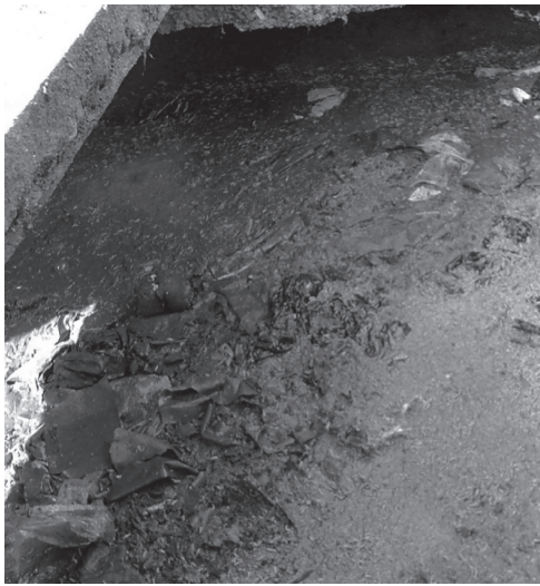
Picture 1: Vault of latrine in Tamale, Ghana. (Note the anal cleansing and other materials that might disrupt vacuum tanker operations)
