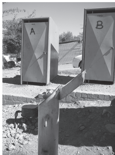
Photograph 3. Flush toilets with pre-paid water tap (in front)
