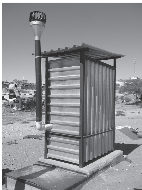
Photograph 2. Dry sanitation with collection chamber (black lid) and rotating self propelled wind turbine extractor
