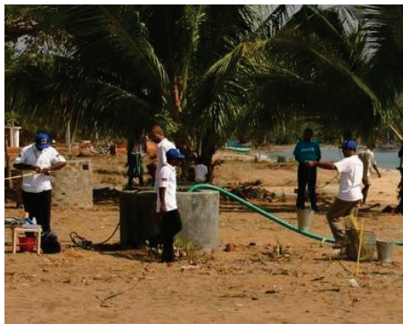
Figure 5. “Controlled” well dewatering operations
