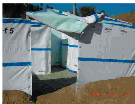
Photograph 2. Looking inside a screened latrine and toilet block
