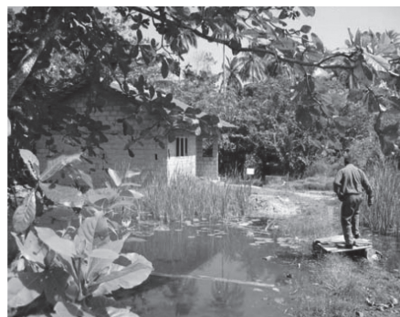
Photograph 2. Water logged marshy land identified for tsunami housing in Kalutara
