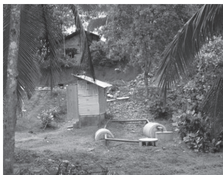
Photograph 1. A Hume-pipe septic tank system used in a transitional camp in Kalutara
