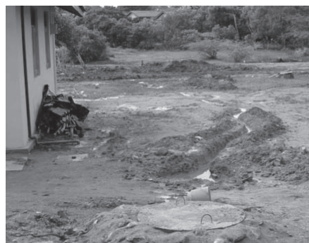
Photograph 3. Failed hume-pipe septic tank and soakage pit system due to lack of soakage resulting in unhygienic conditions in a Kirinda housing scheme
