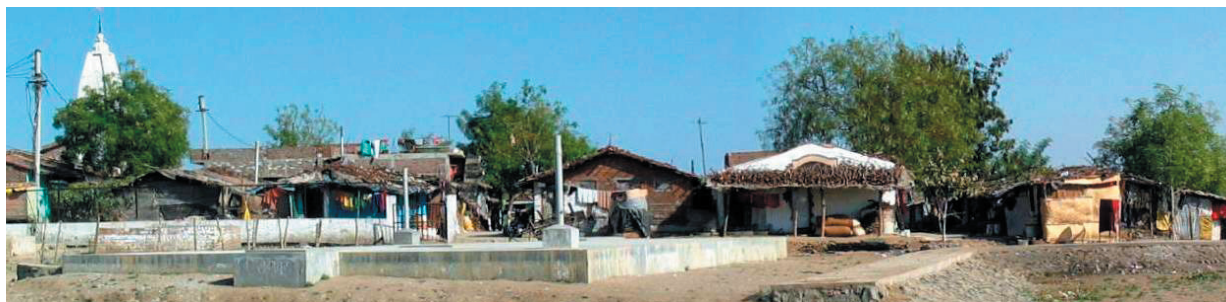
Photograph 1. Sanitation infrastructure (foreground: baffle reactor and pond) at Mahajan Nagar community (background)
