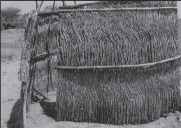
Photograph 4. Superstructure made of grass mats
