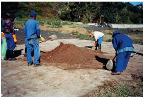
Photograph 2. Mixing the faecal material prior to vault insertion
