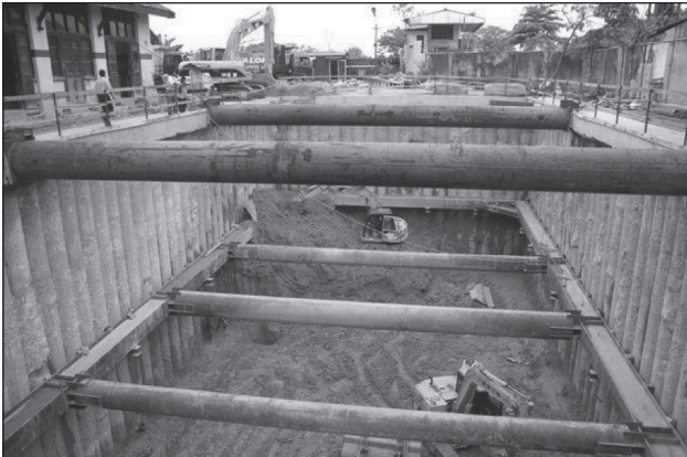
Figure 3. Established cofferdam for construction of the new pumping station
