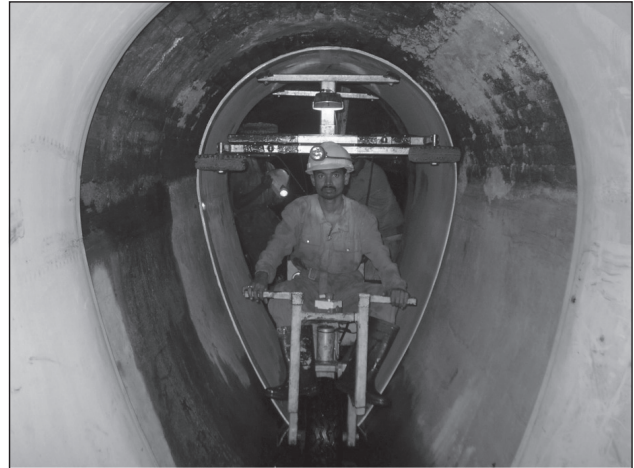
Figure 10. Transportation of GRP inside existing pipeline
